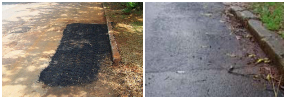
Temporary restoration (left) includes asphalt or gravel patches, hay for erosion control, and other short-term measures. Final restoration (right) may include permanent asphalt patches or repaving, seed or sod in yards, and sidewalk restoration.
