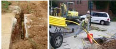
Open cut construction (left) and directional drill installation (right) are the most common methods of completing a replacement project. On occasion a method referred to as "pipe splitting" will be utilized. In this process old abandoned gas pipe will be split and inserted with new plastic pipe.
