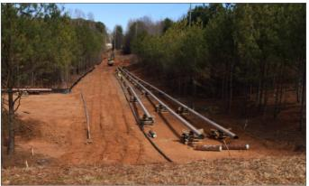
A drill rig is used for boring or directional drilling installation. It hollows out a space below ground that the pipe is then pulled through. Sections or "strings" of pipe are lined up in the easement or right-of-way as part of the installation process. The size of the rig varies depending on the size of the pipe and the length of the section being installed.
